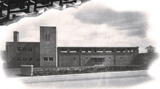
CANTEEN AT No. 1 FACTORY.
