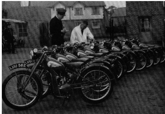
A batch of 125 c.c. two-stroke Royal Enfield motorcycles ordered by the Ministry of Supply on behalf of the G.P.O., for messenger duties, recently came off the production line. The picture shows Mr. Harold Laight, of the Progress Department, checking them over with a motorcyclist from the Redditch Head Post Office. At the request of the postal authorities, the machines were specially equipped with Legshields, Bumper Bars and Duplex Licence Holders.
